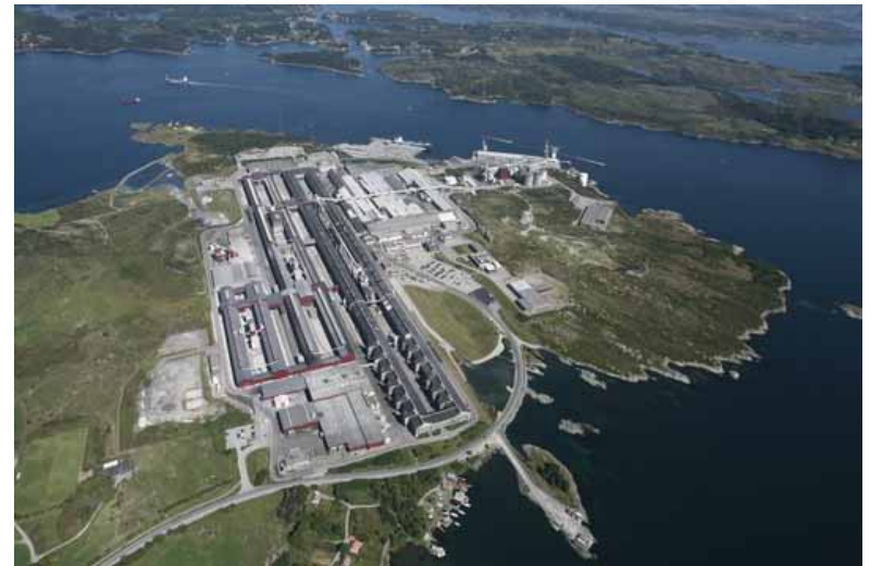
Karmøy Plant, Photo: Tor Alvseike, Hydro
